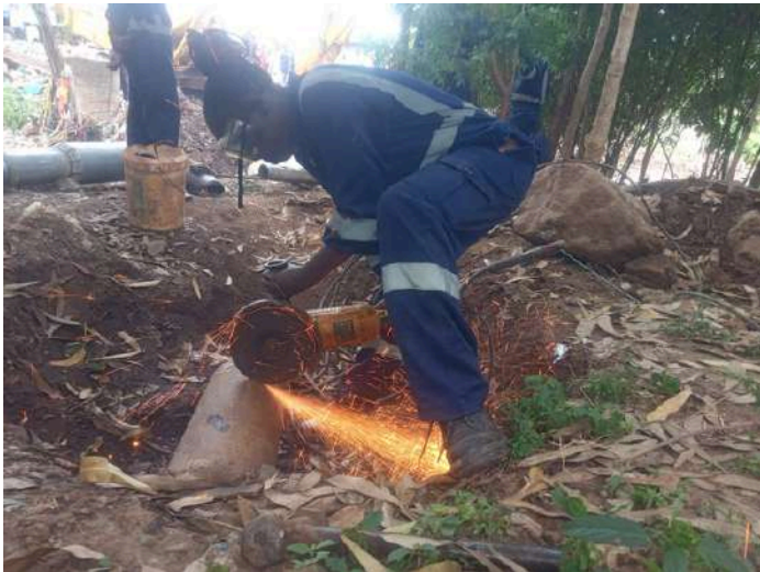
Margaret Wangui reinstating an 8-inch water supply pipeline at Ngomongo Village.
