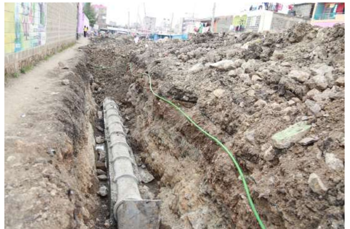
Ongoing construction of sewer line in Mowlem Ward
